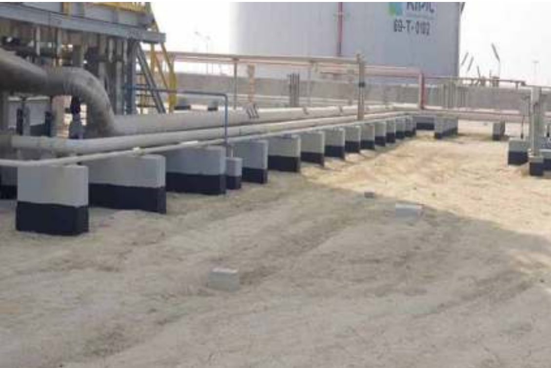
Area A14: Secondary Sleepers Bitumen Painting
