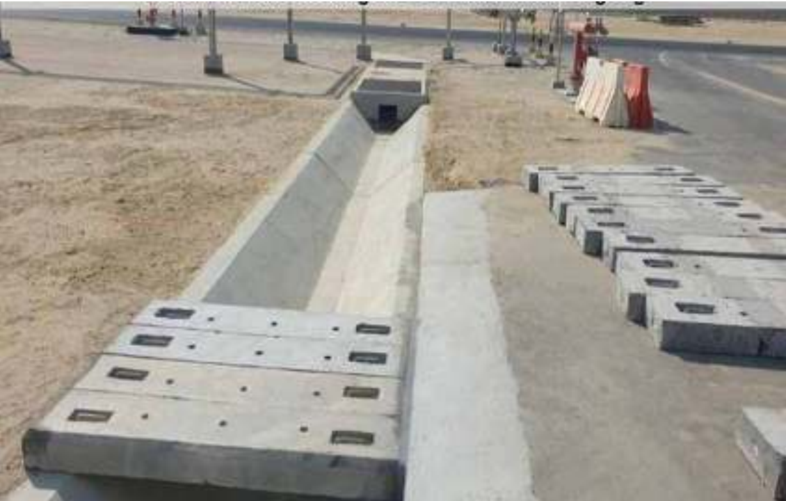
Area A14: Swale Cleaning and Cover Installation
