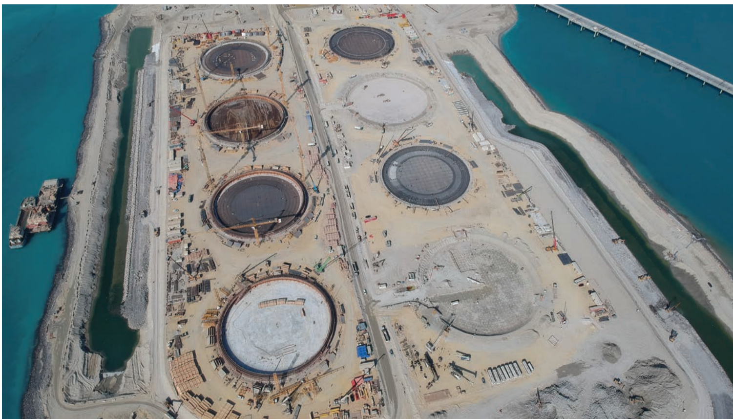
Concrete base at LNGI project
