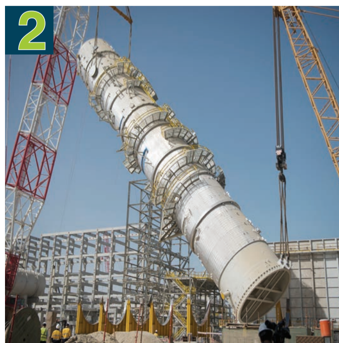
Phases of installing crude distillation column
