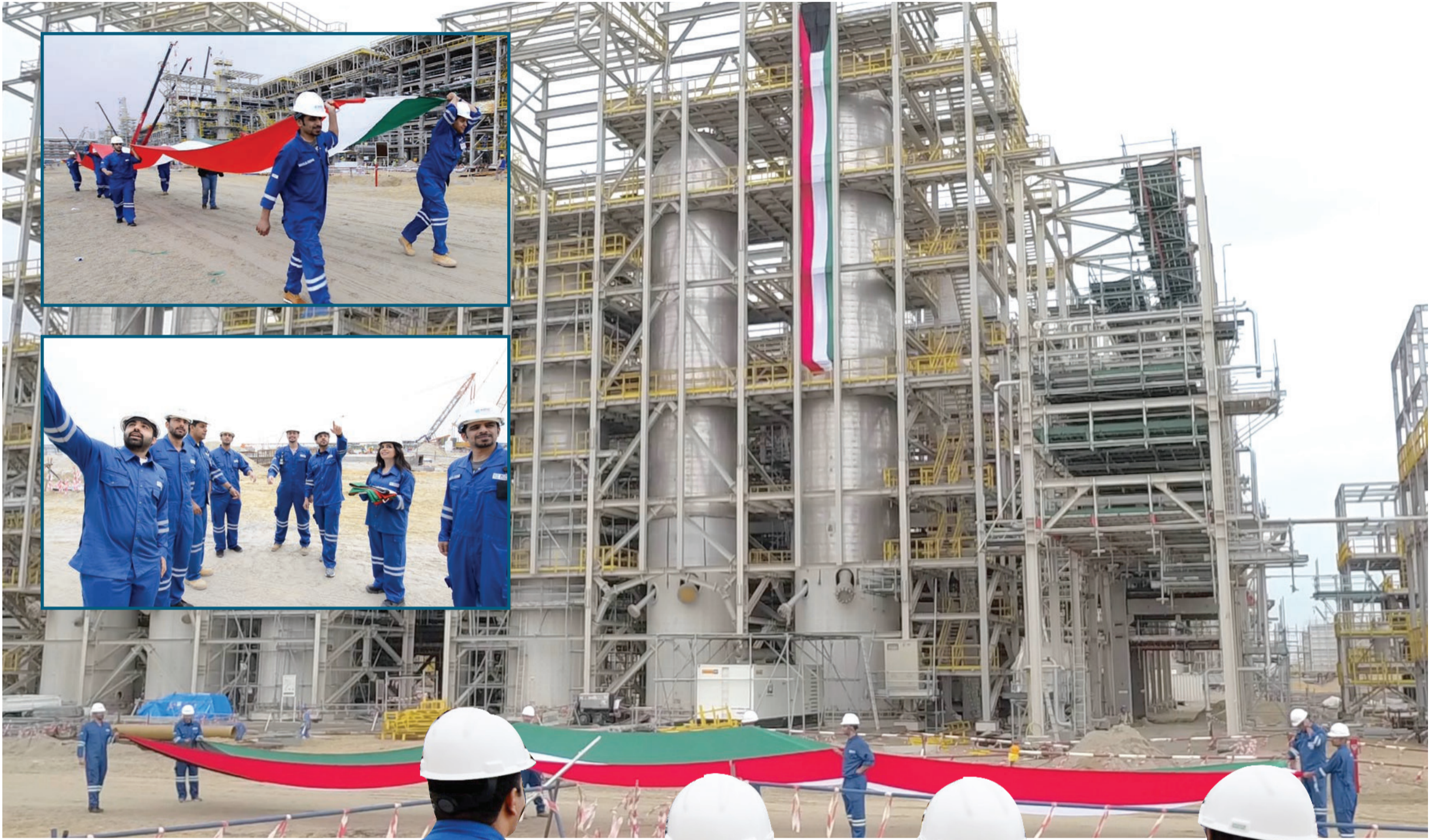
KIPIC's employees carrying Kuwait's flag to be raised over Al-Zour Refinery
