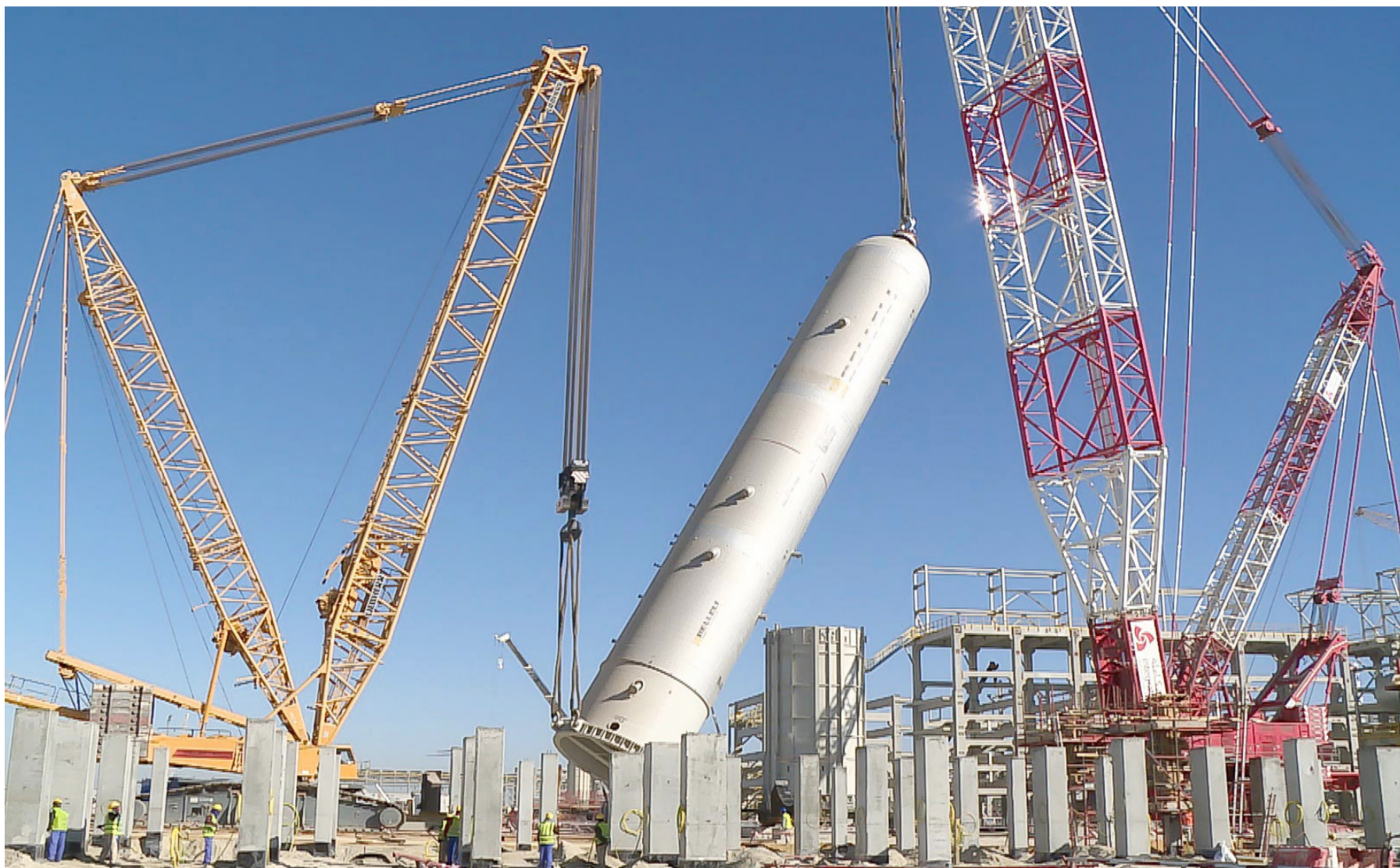
Installation of a reactor at a diesel hydrotreating unit of Al-Zour Refinery's Package One
